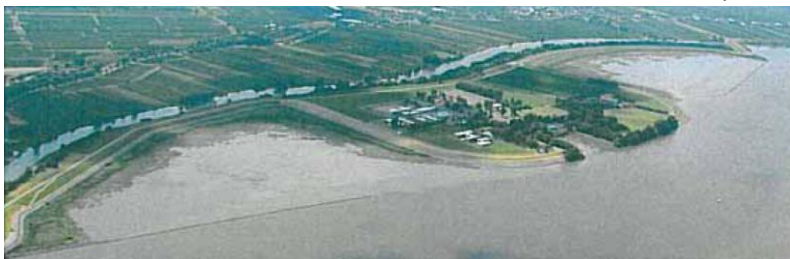
Figure 1: Two created bays at 'Hahnöfer Sand'
