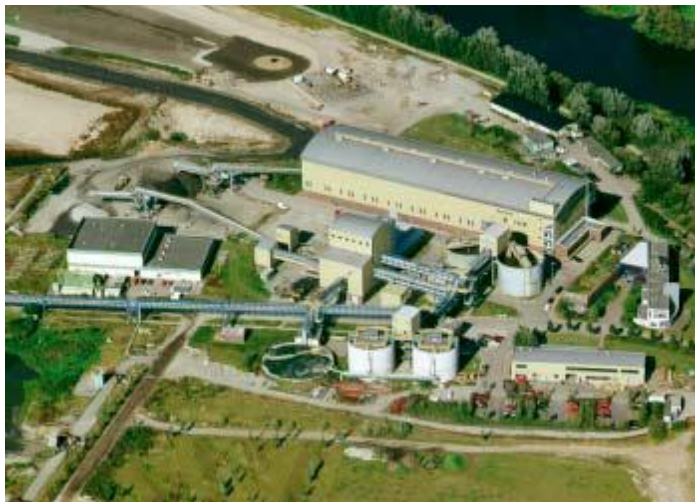
Figure 1 : METHA plant close to Finkenwerder
