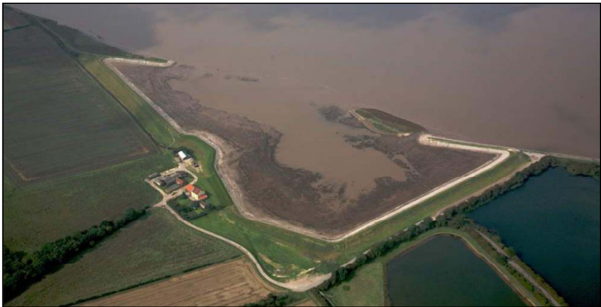
Figure 3: Aerial view of site in December 2006 (5 months post realignment) (taken by ABP)
