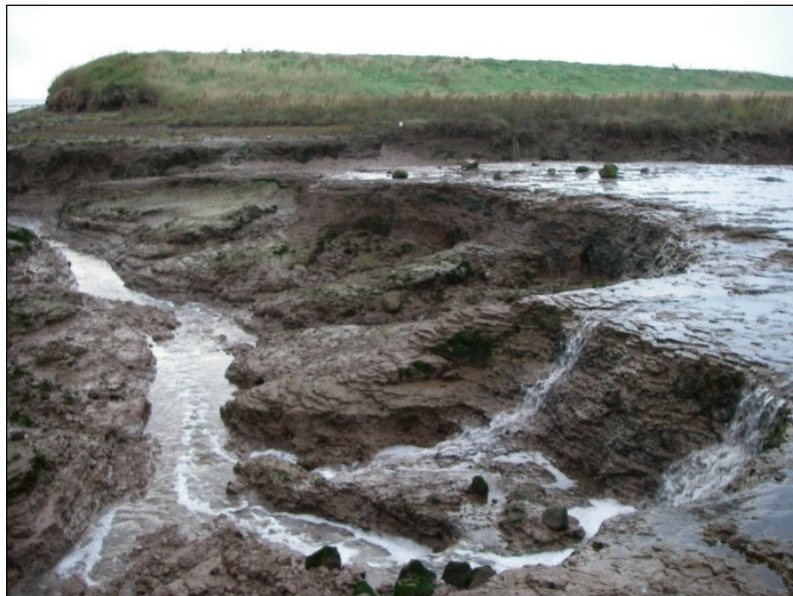
Figure 7: Creek through southern breach eroding mudflat area (S.L. Brown, 2008)
