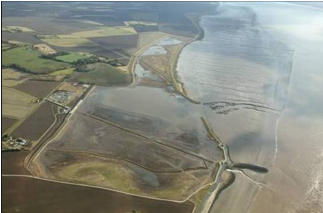
Figure 2: Aerial photograph of project area (right) after the embankment breaches (October 2003)
