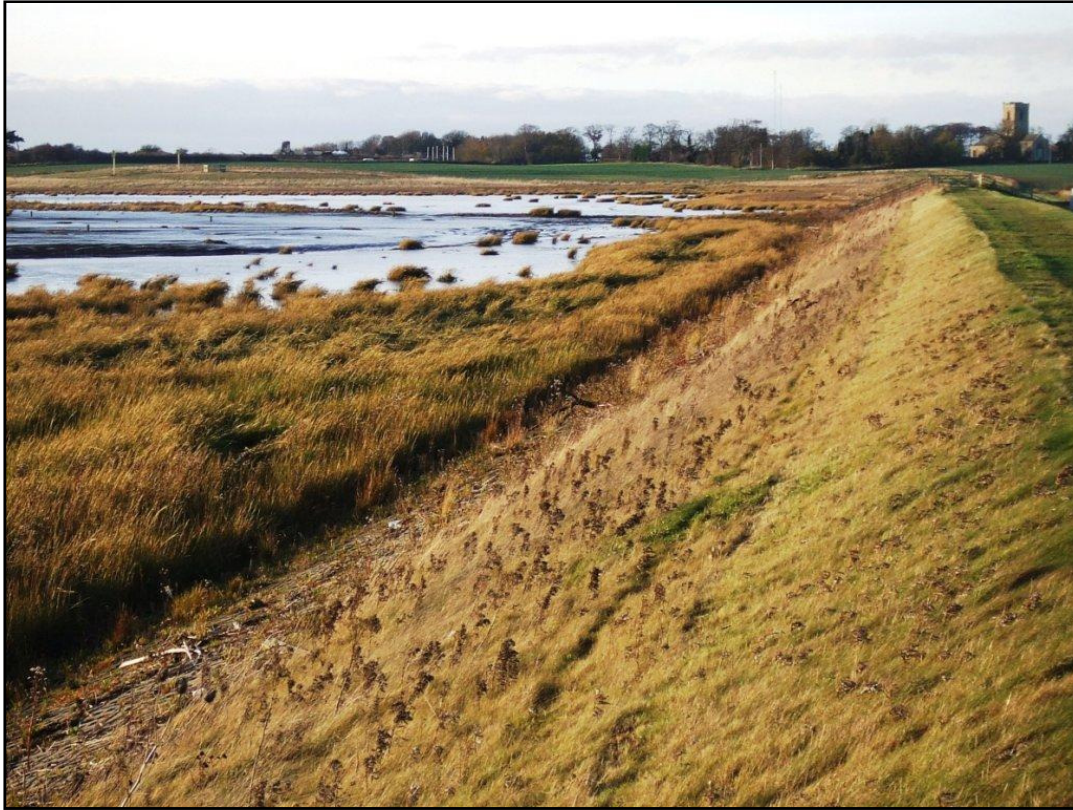
Figure 4: View of embankment (taken by Nigel Pontee, Halcrow)
