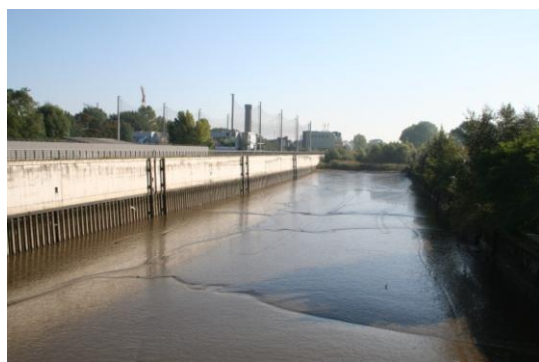
Figure 1 Mudflats in the channel 'Haken'
