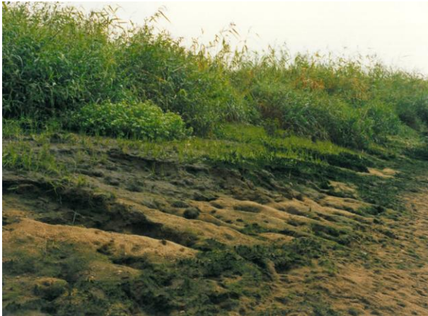
Figure 3: View of the erosion of the slope
